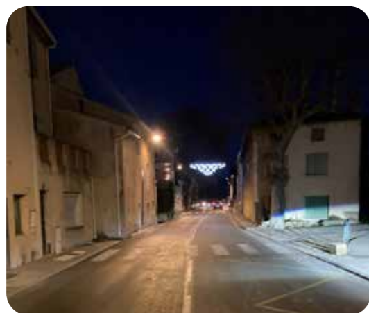
ROUTE DE VALREAS ECLAIRAGE LED
